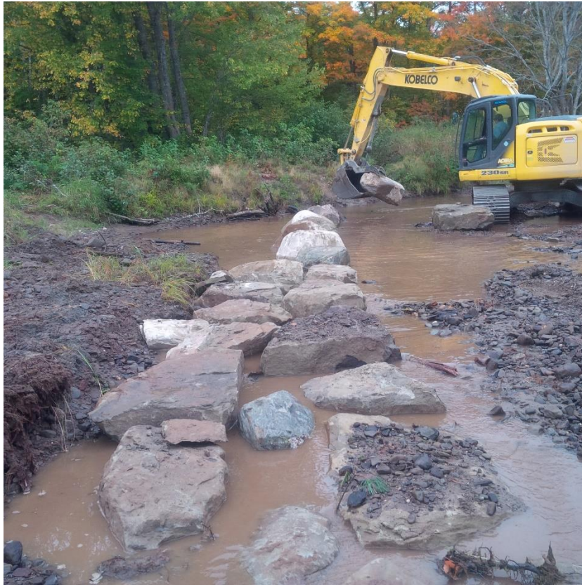
Rock weir installation.
